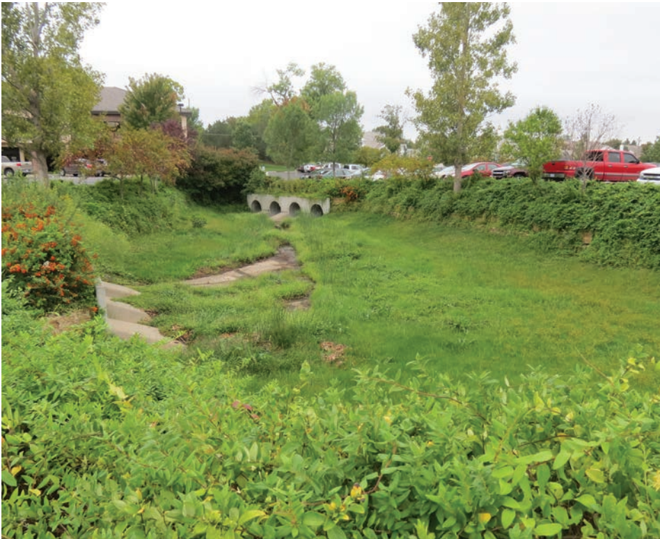
Figure 11. One of a series of water retention ponds that hold runoff water from roofs and parking lots of a business complex that was originally a wooded area. The inlet and outlet culverts control the rate of flow to the receiving downstream drainage area. The retention ponds are vegetated with wetland plants. (Photo courtesy of Danny H. Rogers.)
