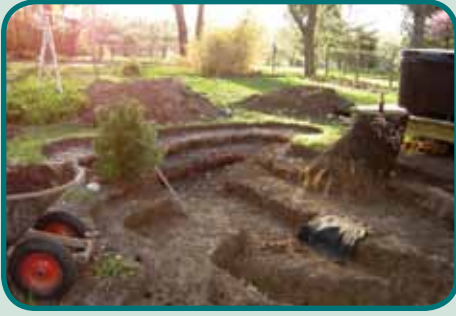
Digging the hole
