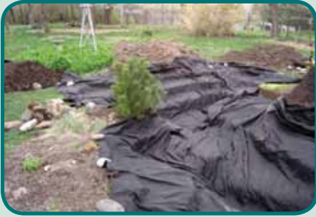
Laying the liner
