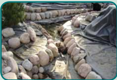
Placing the large rocks
