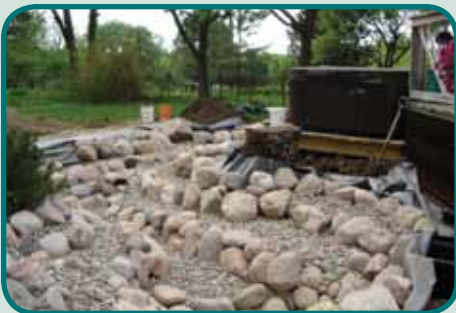
Placing the small rocks
