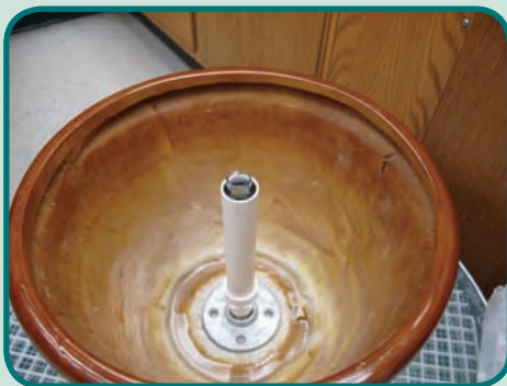
Figure 16. Assembled plumbing in pot.
