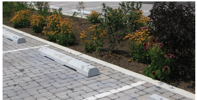
Figure 8. Permeable pavement (credit www.epa.gov).
