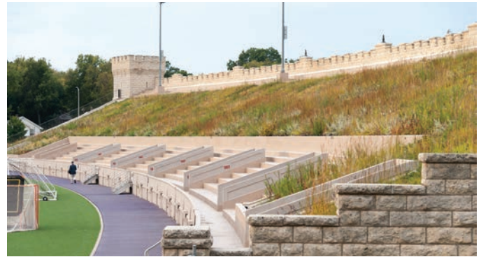
Figure 7. Green roof at Kansas State University Memorial Stadium.
