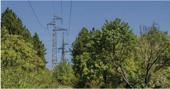
Figure 8. Structural inspection and maintenance is made easier with vegetation control.
