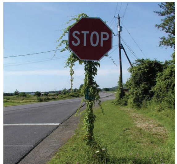
Figure 13. Woody and herbaceous vines can persist along the edge of the right-of-way and impact signs. Photo: Dan Wixted, Cornell University
