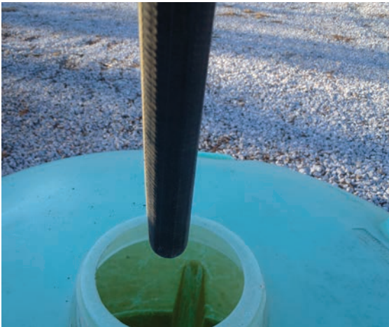
Figure 1. An air gap prevents herbicide solution from contaminating water sources. Photo: Jan Hygnstrom
