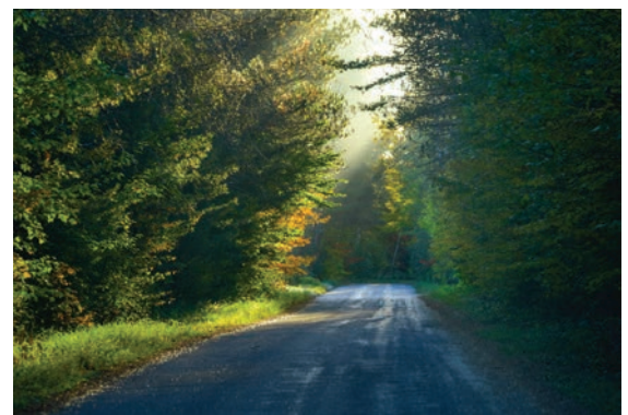
Figure 3. Trees obstructing the view of the roadway.
