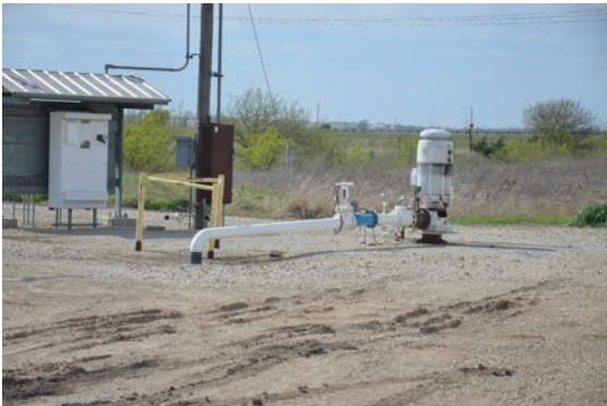
Figure 14. Vegetation control allows for pipeline inspection and maintenance. Photo: Frannie Miller
