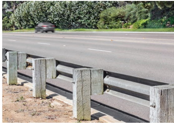
Figure 1 Guide rails must be kept visible to motorists and maintained.
