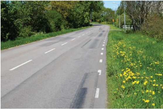
Figure 4. Control of tall weeds along the roadside helps move water off the highway.
