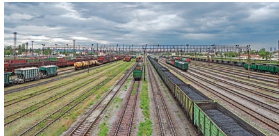
Figure 10. Vegetation in yards presents a hazard to railroad employees.
