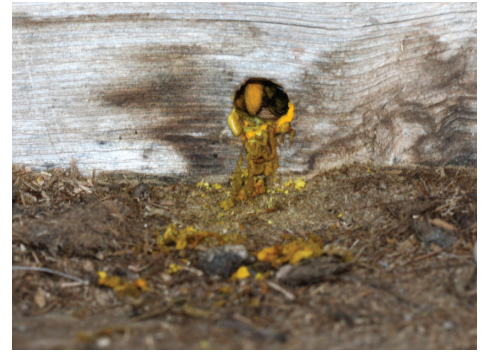
Figure 5: Carpenter bee tunnel entrance with sawdust and pollen trail
